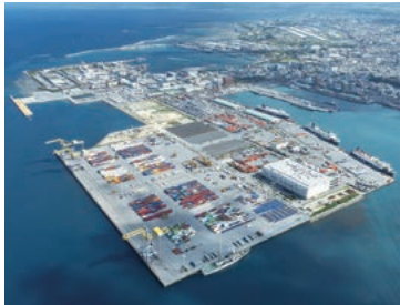
Naha Port Public International Container Terminal
