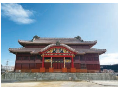
Shuri Castle Main Hall under reconstruction (November 2025)
