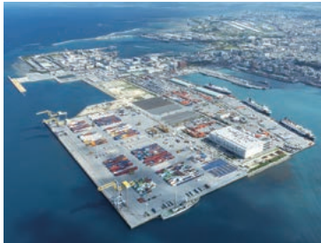
Naha Port Public International Container Terminal
